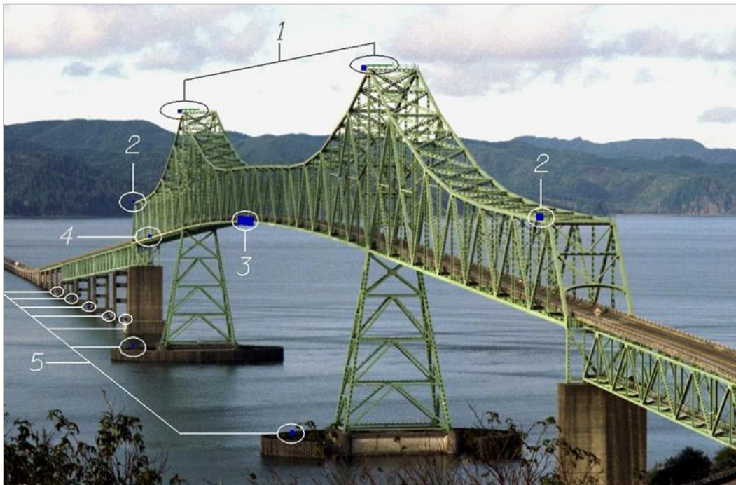
Figure 6: Locations of the five different types of solar lights on the Astoria-Megler Bridge Photo credit: ODOT
