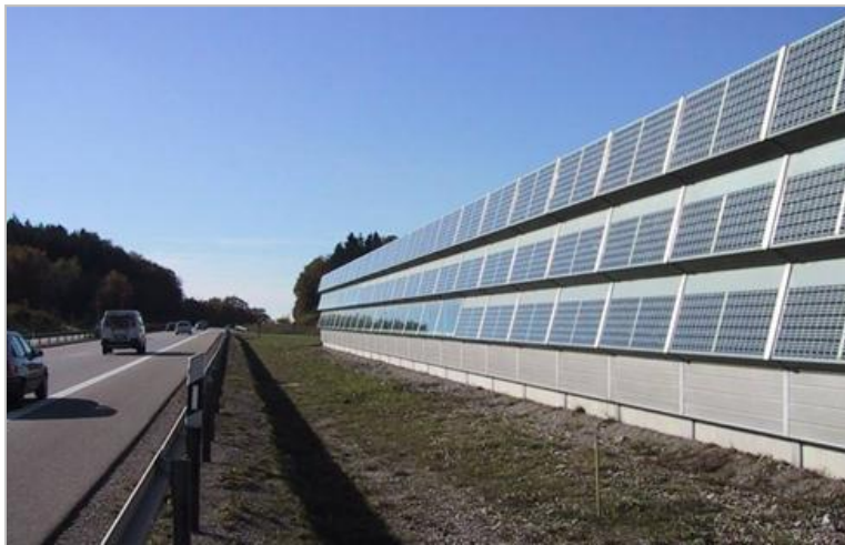
Figure 2: PV system mounted on a noise barrier in Europe
