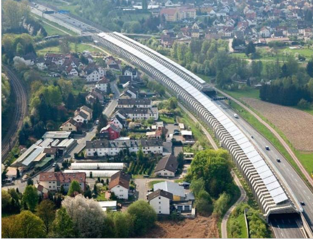
Figure 3: The German Unity Motorway Planning and Construction Company constructed a 2.8-megawatt (MW) solar array on the roof of a 2.7 km long noise-barrier tunnel on the A3 highway near Aschaffenburg, Germany.
