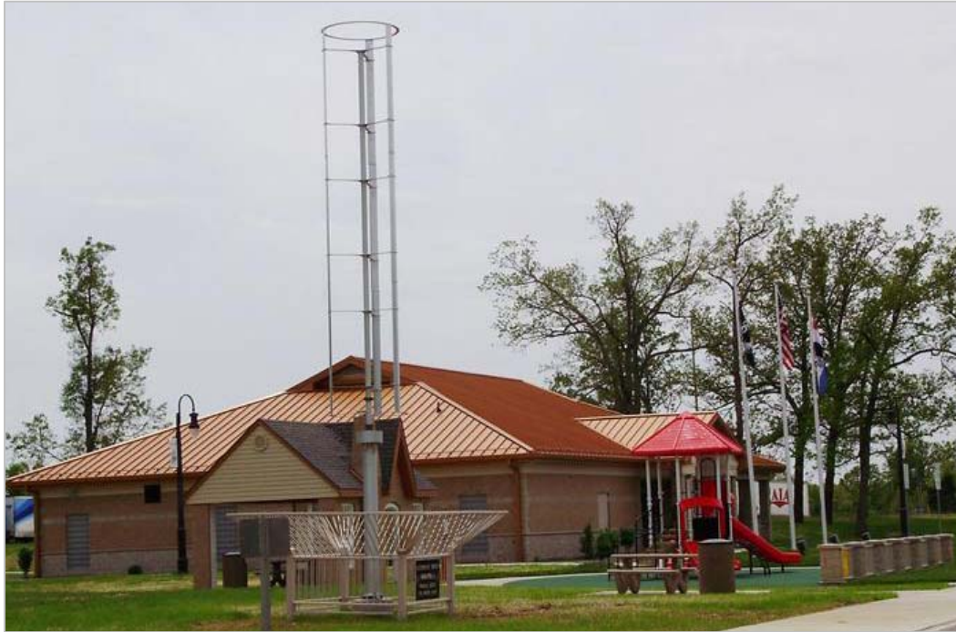
Figure 11: One of two, 1.2 kW wind turbines (one in each traveling direction) installed at Missouri DOT's Conway Missouri Welcome Center on I-44 . The wind turbines power the lights over the information counters.
